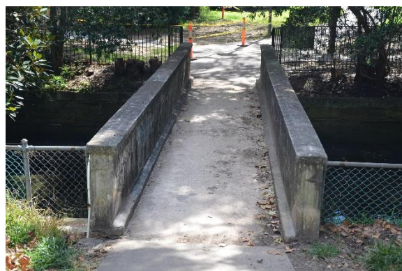
Figure 2.24 An early–mid twentieth-century footbridge over the stormwater channel in the south of the park. (Source: Ari Anderson, 2021)
