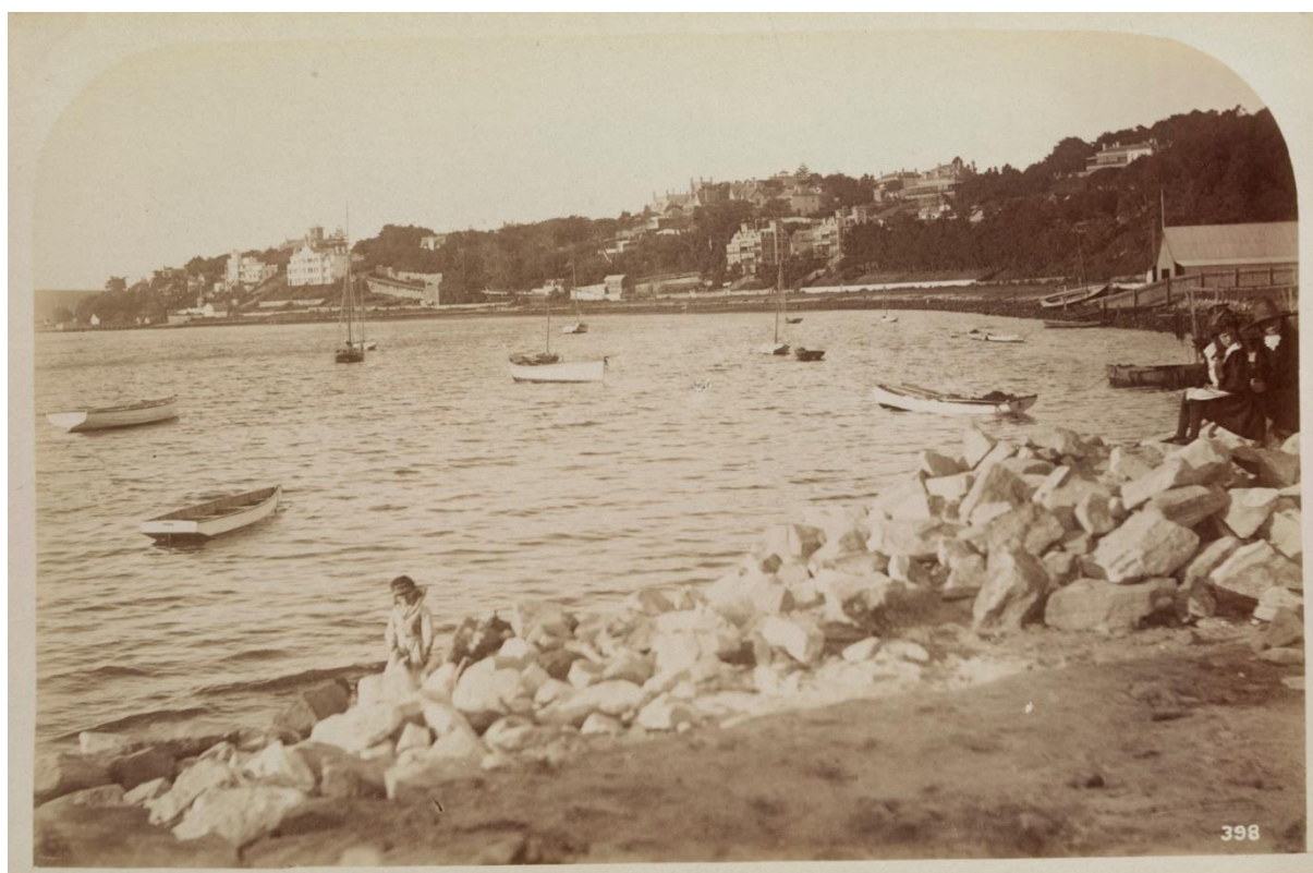
Figure 2.85 The study area’s ballast dyke seawall, c1890s. (Source: State Library of Victoria, H39359/45)
