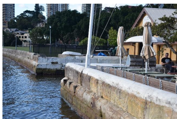
Figure 2.50 The seawall and gap for the RANSA slipway. (Source: Ari Anderson, 2021)
