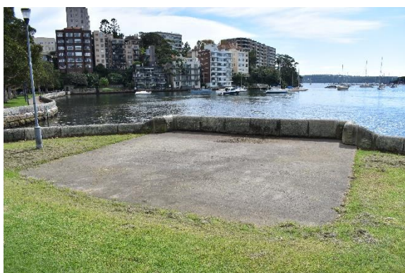
Figure 2.29 An area of hardstand concrete with a modified area of the seawall, below which is a separate outlet.
