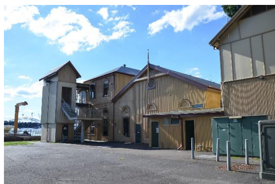
Figure 2.46 The former HMAS Rushcutter Drill Hall. (Source: Ari Anderson, 2021)
