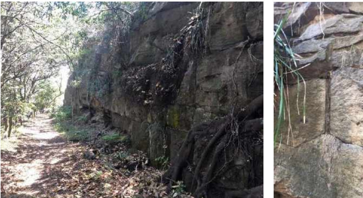
Existing track along the proposed route of path with visible signs of sandstone cutting
