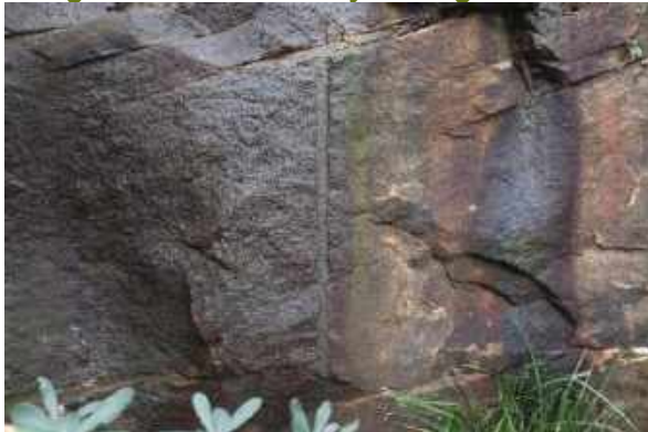
Figure 5-15. Example of remnant drill marks along the former tramway cutting.
