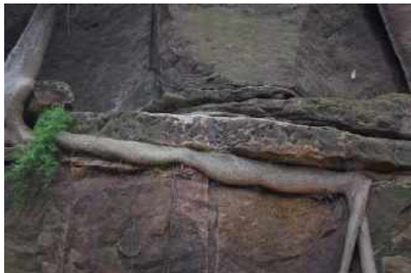
Figure 5-14. Example of remnant chisel marks along the former tramway cutting.
