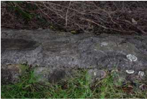
Figure 5-27. View west looking down slope from the former tramway showing a concrete and stone retaining wall.
