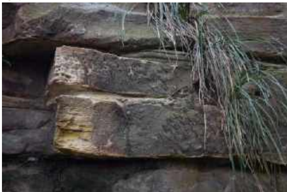
Figure 5-13. Example of remnant chisel marks along the former tramway cutting.
