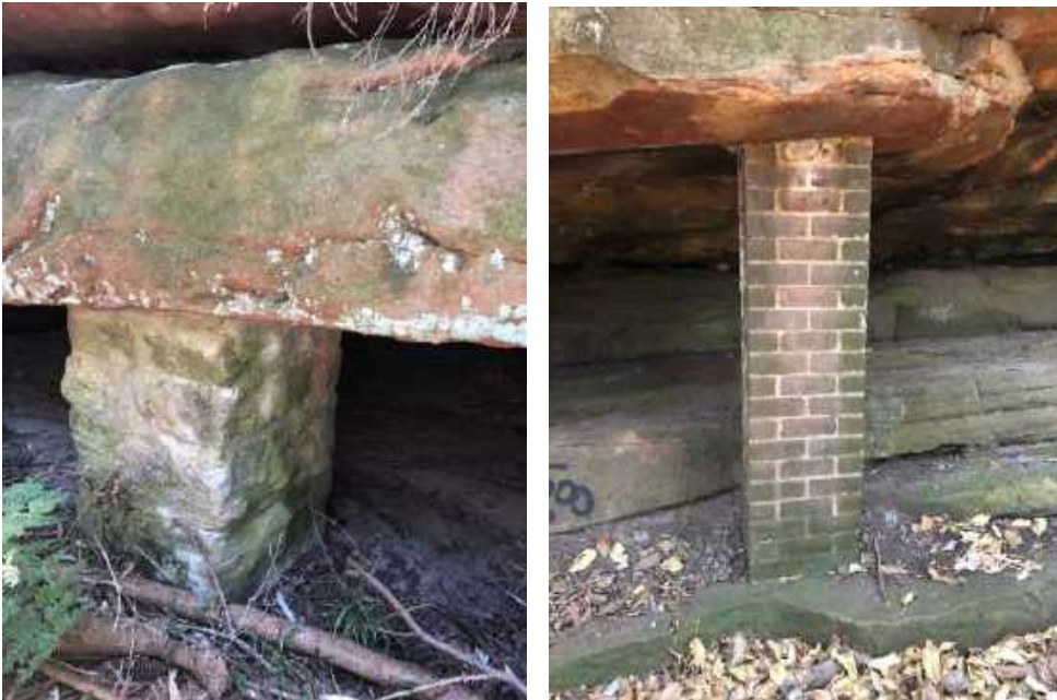
Example of piers constructed to provide support to natural rock shelves
