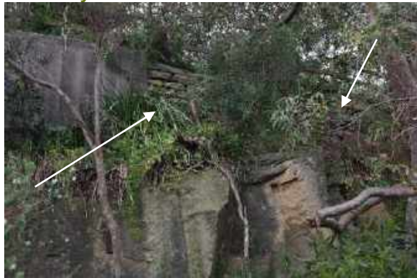
Figure 5-28. View east towards to tramway route from Gap Road showing examples of concrete and sandstone retaining walls along the northern end of the former tramway route.
