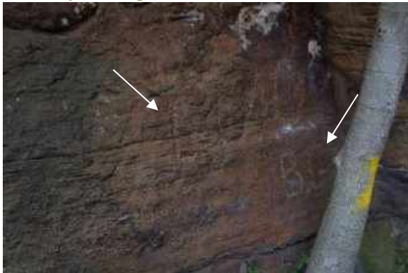
Figure 5-19. Example of graffiti (L.U and B.G) engraved and painted onto the northern end of the tramway cutting.
