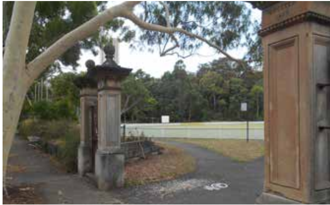
Figure 22. Sandstone posts bearing the name "Hampden Park" flanking the entrance to Trumper Park off Glenmore Road
